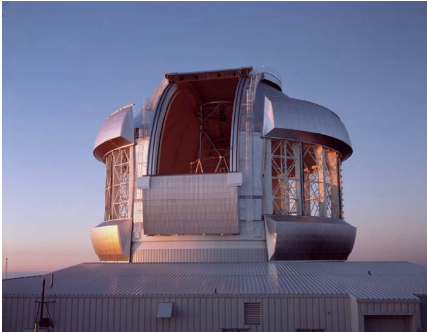
Figure 1. Gemini enclosure with large ventilation gates to allow natural ventilation with ambient air
