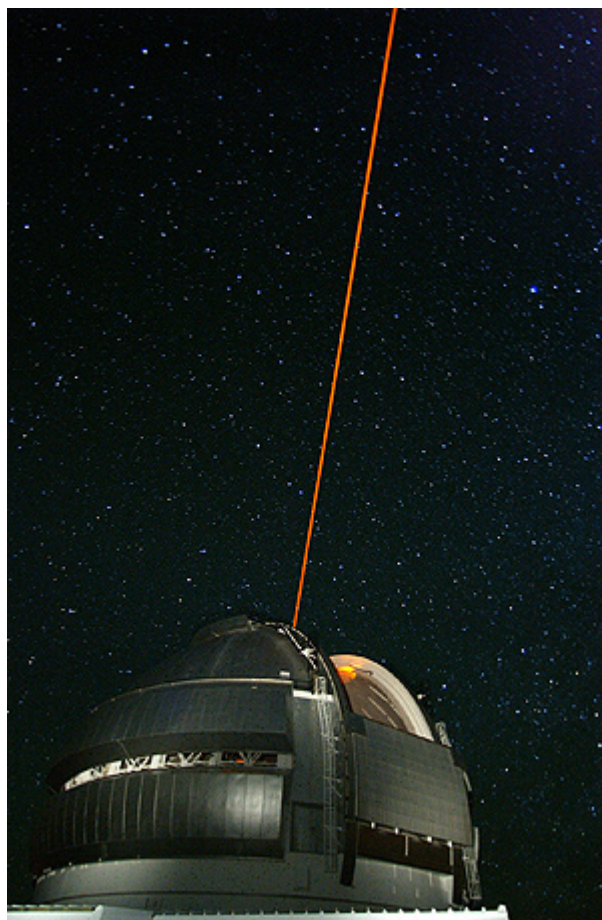
The laser-guide-star beacon at Gemini North. Laser-guide-star adaptive optics will be offered for the first time in semester 2006B. (Image Credit: Gemini Observatory)
