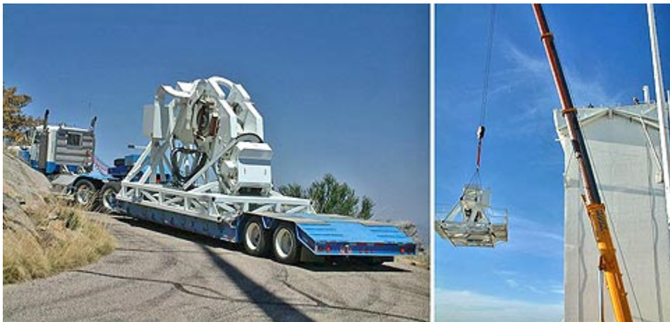
Figure 1. The SOLIS mount arrived on Kitt Peak and was lifted to the top of the old Vacuum Telescope tower in April. (Photographs by David Jaksha.)
